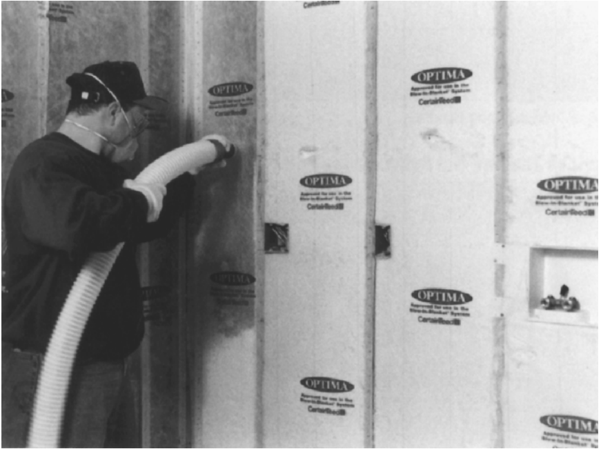
Figure 9.7 Installing the blow-in-blanket system. (CertainTeed)
